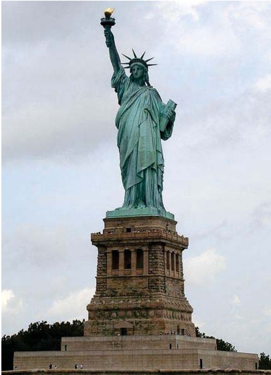
Figure 7.2: After an initial green layer of copper oxide formed on the surface, the copper of the Statue of Liberty has not corroded further.
